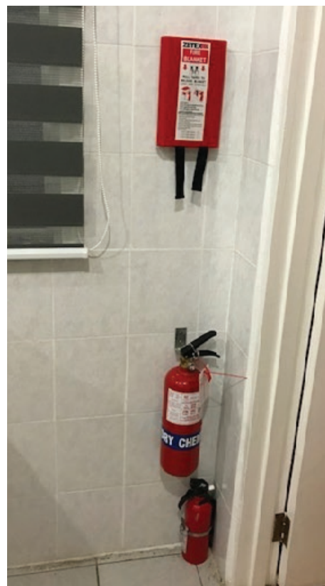
This picture shows an easily accessible and clearly visible fire-extinguisher and fire blanket in the kitchen.
